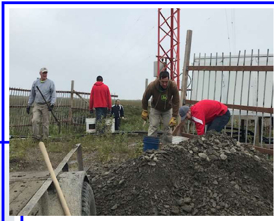
The Vista Team spread a lot of gravel bucket by bucket to level the ground around the center tower
