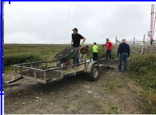
The Vista Team spread a lot of gravel bucket by bucket to level the ground around the center tower
